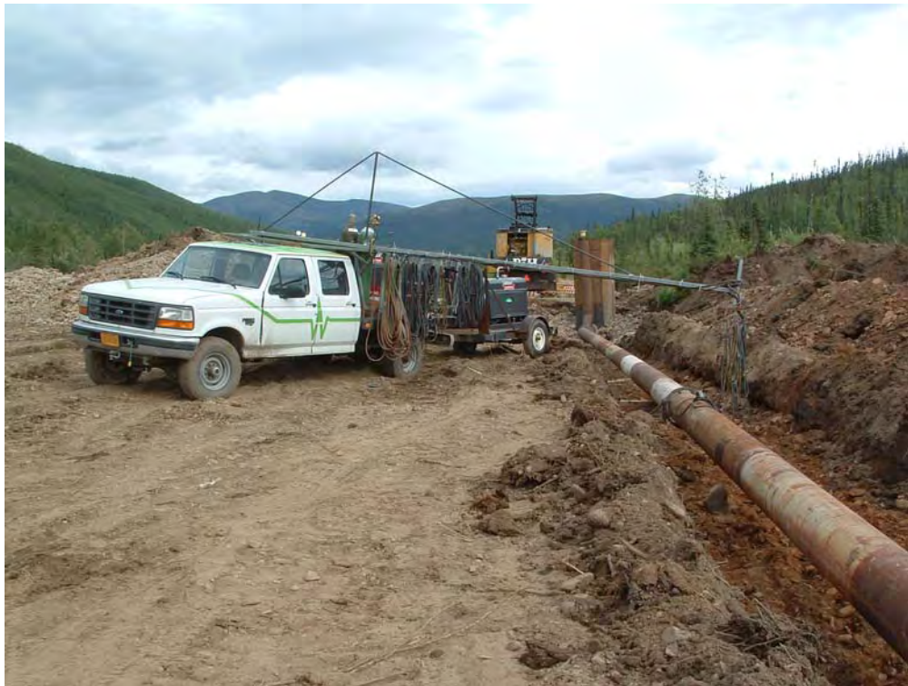
Figure 11. Installation of 16in Cold Water Pipeline, July 2006
