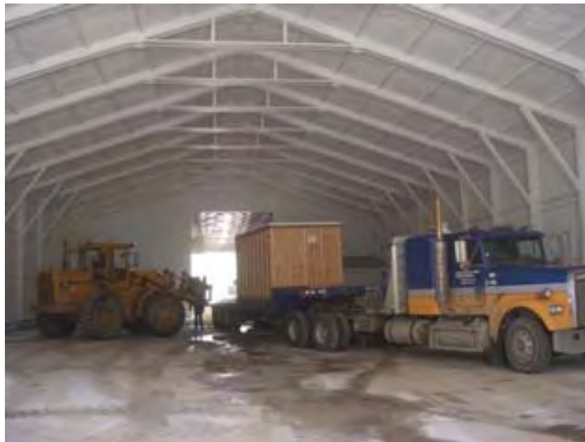
Figure 10. ORC unit delivered to Power Plant building
