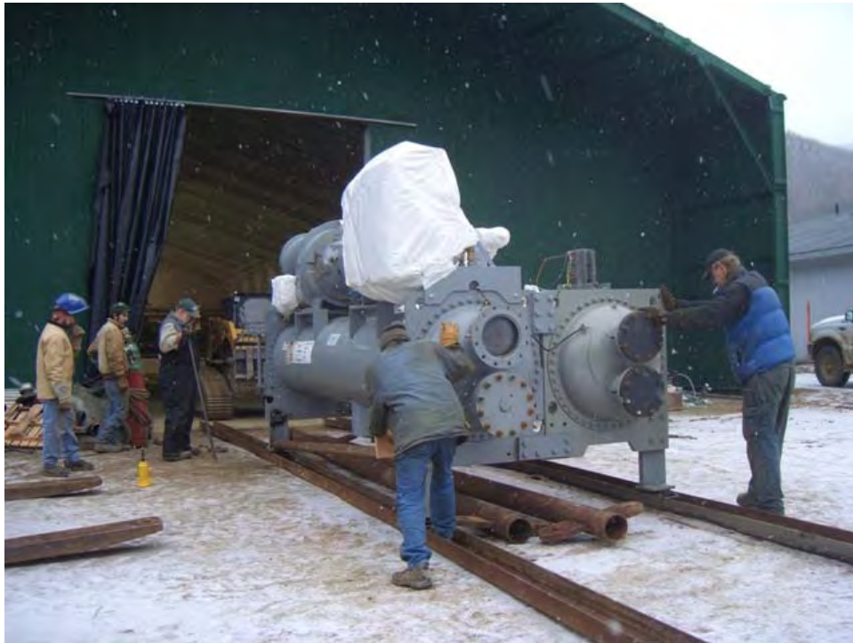
Figure 21. Moving ORC #2 into the Power Plant Building
