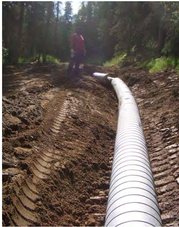
Figure 17. Installation of Hot Water Supply Pipeline
